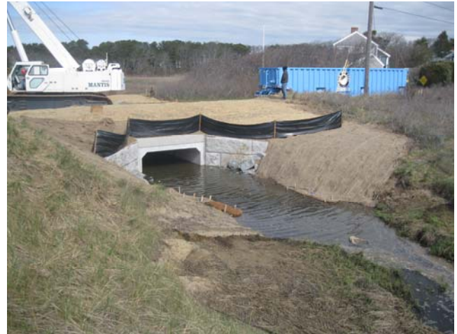
A new culvert in Harwich, Massachusetts
