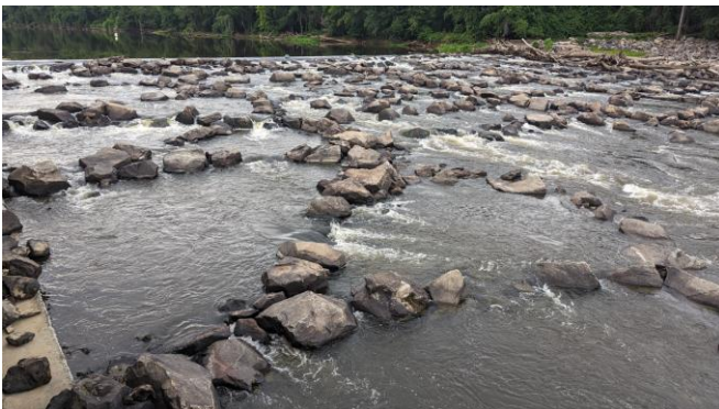
The modified design of the nature-like fishway at lock and dam 1 on the Cape Fear River. Photo credit: Aaron Bunch
